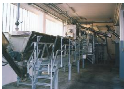
Picture 2: Washery with output 1 t/h. Under construction
