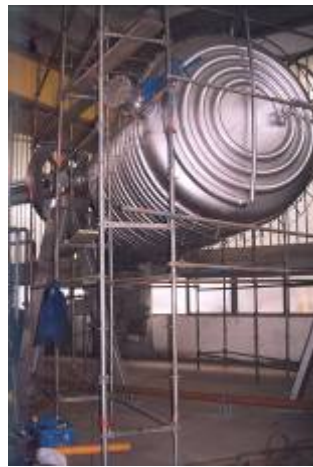
Picture 6: Vacuum crystallization equipment, installation
